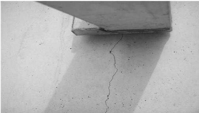
Crack in reservoir (top) and KIS treated (below)
